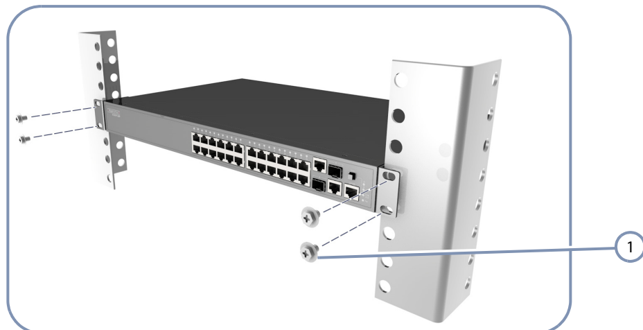
Figure 9: Installing the Switch in a Rack
