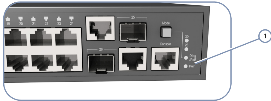
1 System Status LEDs.
